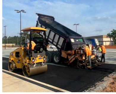
The pickleball courts are making great progress! The courts will need to cure for 30 days before the contractor can stripe the courts. Fencing and gates will be installed during that time. Lights have passed inspection and sidewalks have been installed as well.
