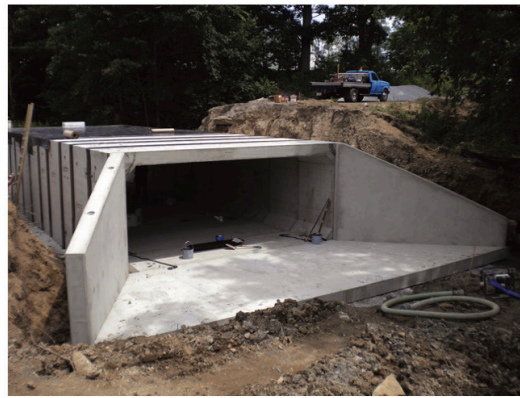
Culvert Replacement
