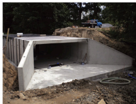
Culvert Replacement
